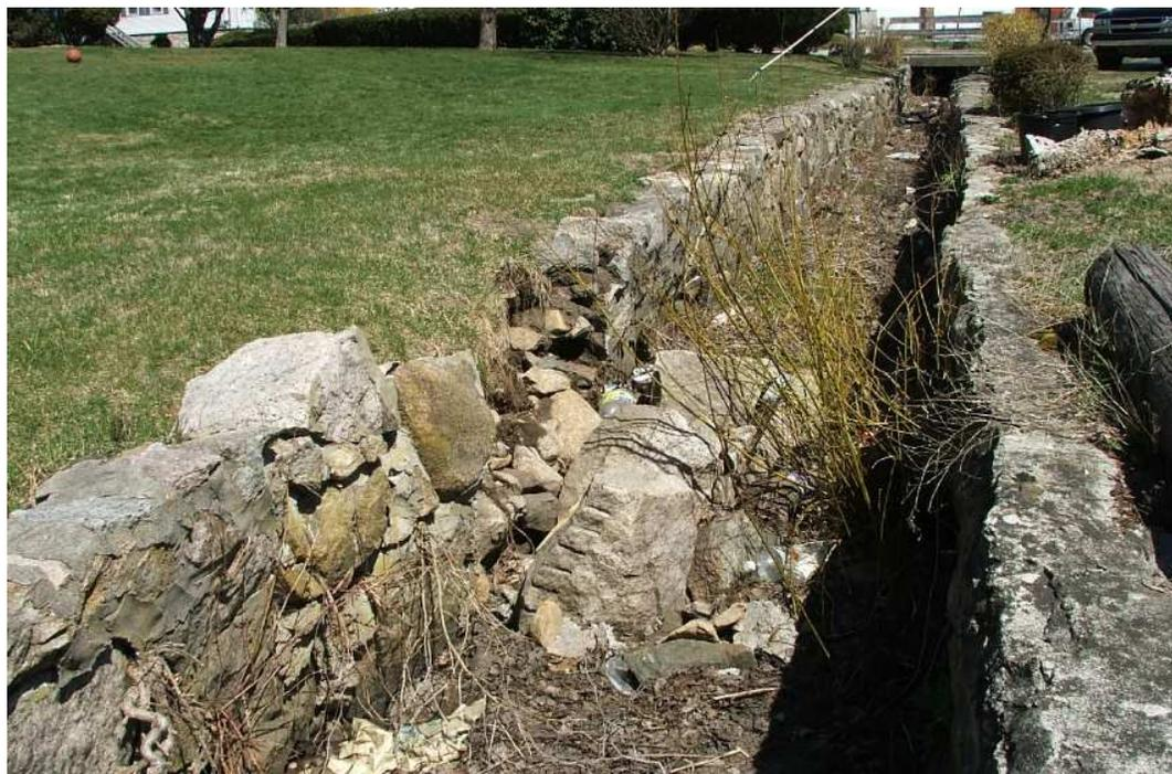
**Photo 3. Failure of Godfrey Brook Channel Stone Walls (2006)**
