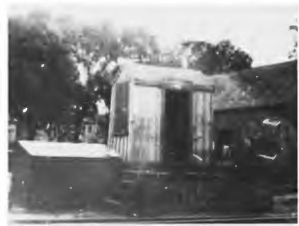
A rare photograph of the lever house in the Boston and Albany yard. Beach and Mt. Pleasant street gates were operated here. Box at left held coal for gateman's stove inside the small building.
