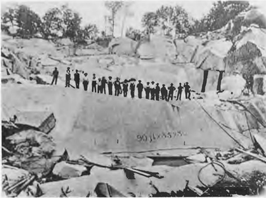
This large pink granite slab was quarried in Milford. It weighed 8000 tons and measured 90 x 35 x 30 feet.
