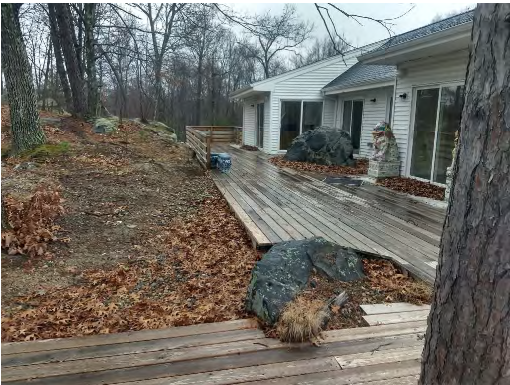
Photo 6: Completed deck on rear side of building, 11/30/2020
