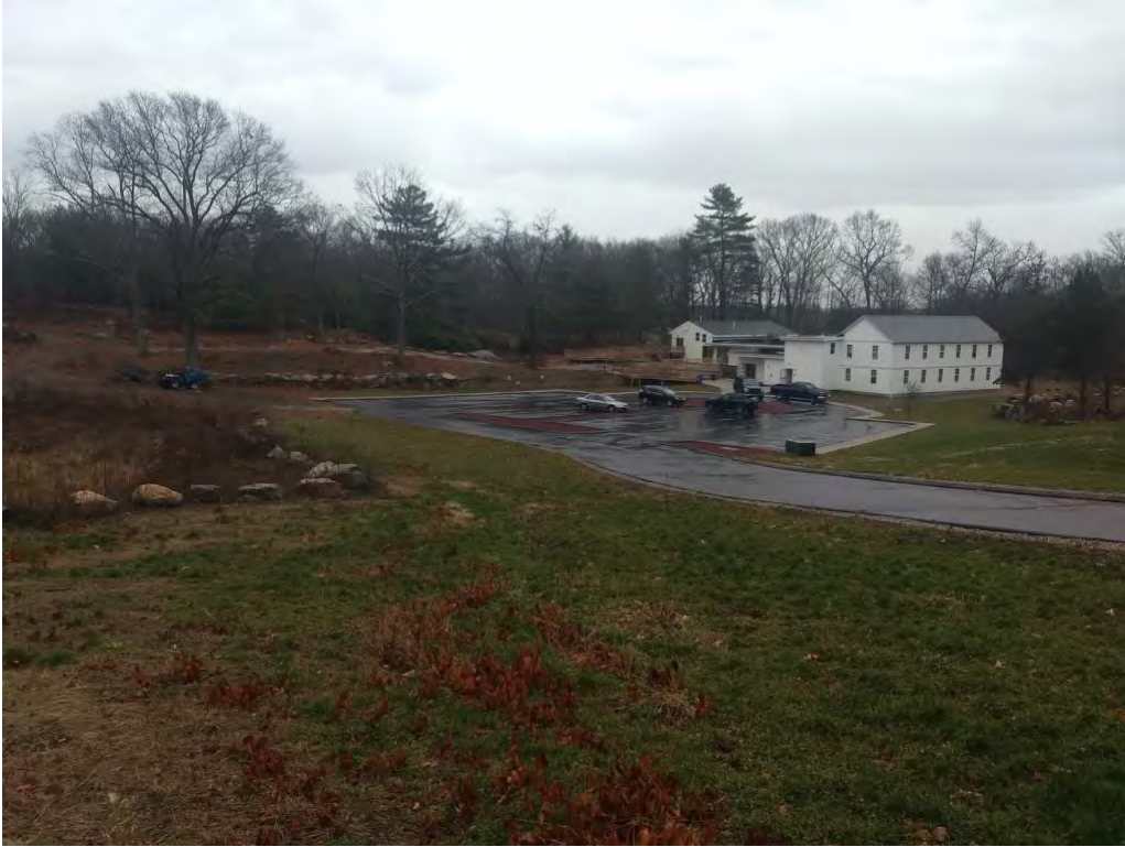
Photo 2: Completed Parking Lot, 11/30/2020
