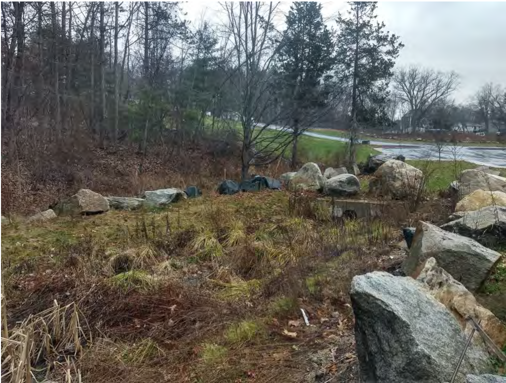
Photo 3: Completed Water Quality Swale, 11/30/2020
