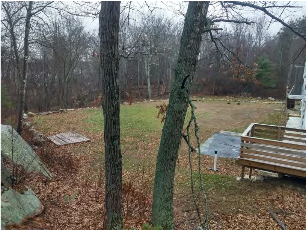
Photo 5: Completed back side of building, 11/30/2020
