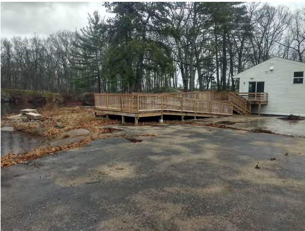
Photo 8: Completed decks around previous patio and paved area, 11/30/2020
