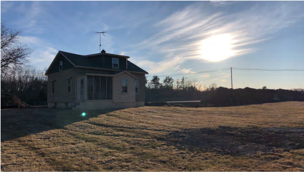
Photo 1: The existing single-family home on Lot 25 stands in the middle of a vast lawn.
