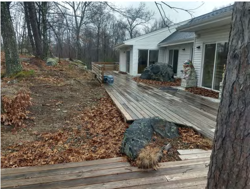
Photo 6: Completed deck on rear side of building, 11/30/2020
