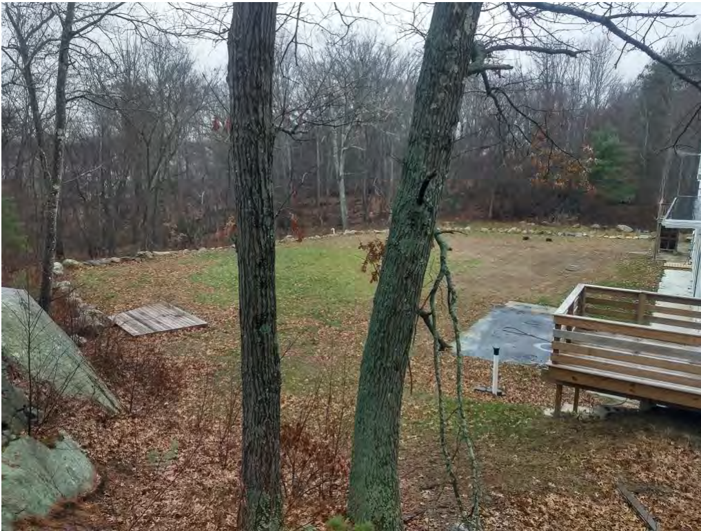
Photo 5: Completed back side of building, 11/30/2020
