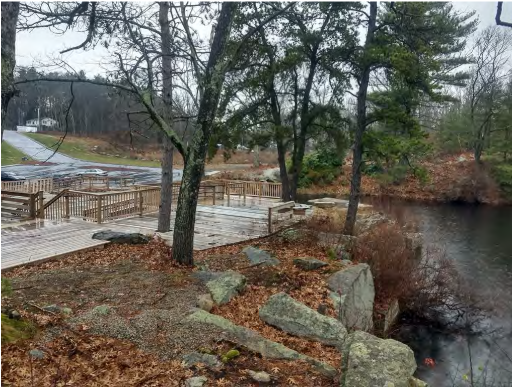
Photo 7: Completed deck on rear side of building, 11/30/2020
