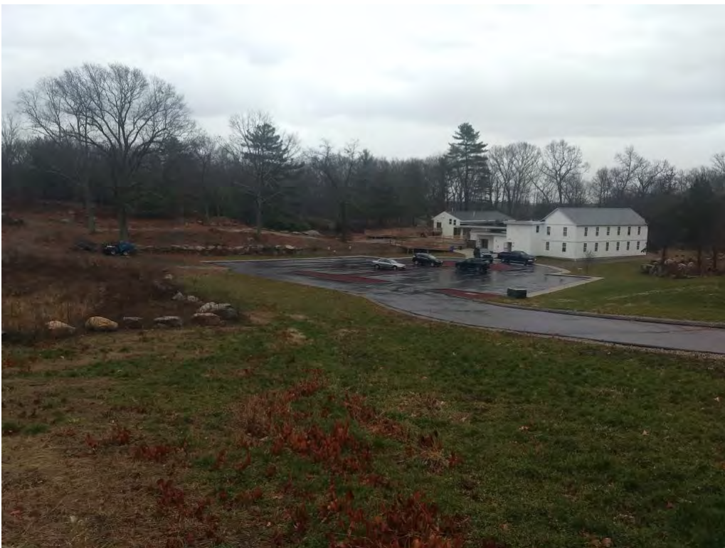
Photo 2: Completed Parking Lot, 11/30/2020
