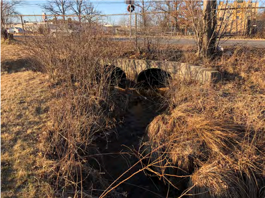
Photo 2: The stream discharges from the double piped culvert below Medway Street. The stream flows through the lawn and eventually enters a narrow grove of woody vegetation on Lot 23C.
