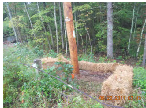
FIGURE 2: ALT. STRAW BALE APPLICATION
