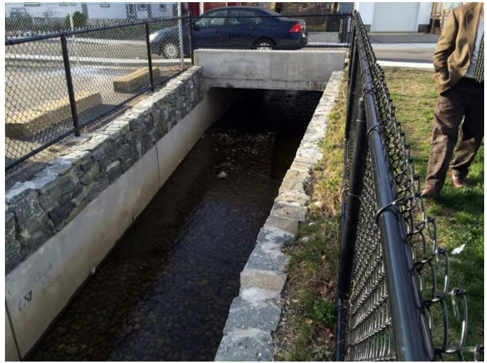
Godfrey Brook Culvert Replacement at Church Street (HMGP Grant #1813-22)
