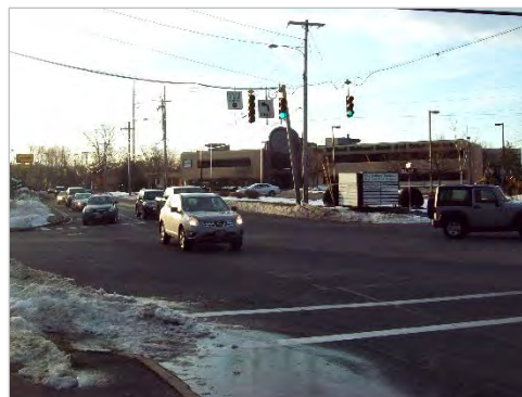
Image 14: Ponding on Fortune Boulevard at Intersection
