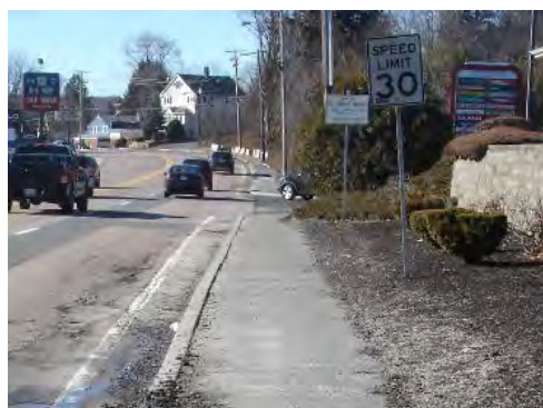
Image 8: Vegetation Obstructing Sight Lines on Northeast Corner of Quarry Square West Driveway Intersection (Looking West Towards Driveway)
