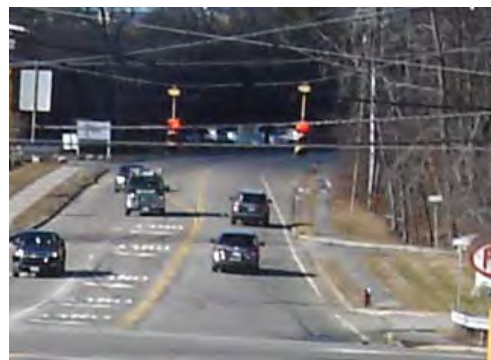
Image 16: Utility Lines Obstructing View of Northbound Signal Heads
