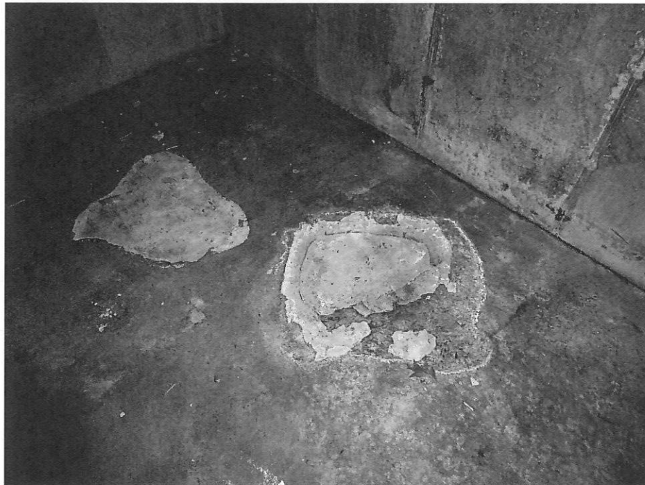
Spalled patches at top of slab-on-grade in Room 101.
