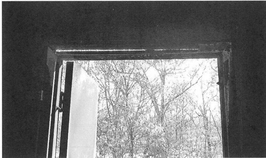
Severely corroded door frame in Room 300.
