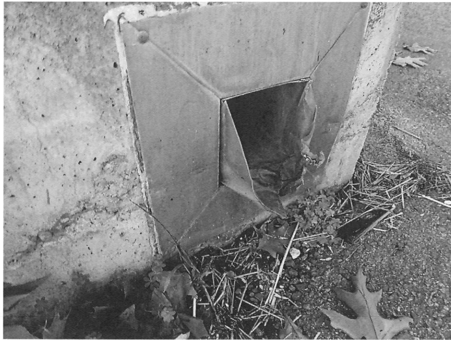
Damaged sheet steel at ground floor scupper opening.
