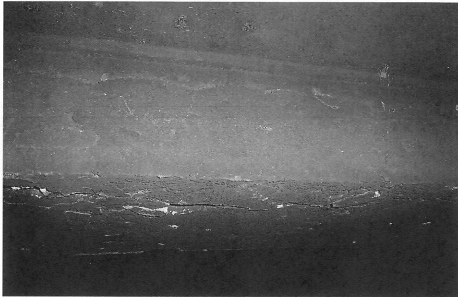
Severely delaminated and cracked beam at underside of high roof slab.
